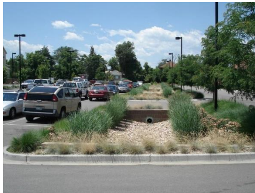
Figure 16-3-3-7. Examples of Bioswales
